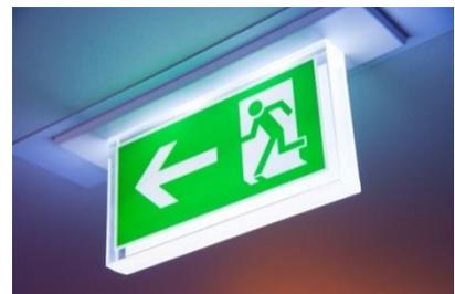
The objective of safety lighting is to enable personnel to reliably stop potentially dangerous work processes and avoid hazardous situations in the event of a general power failure, to get to a place at which an escape route can be clearly recognized as such and to use it in order to safely exit the building or leave the area. In contrast to this, stand-by lighting makes it possible to continue all necessary tasks in an unchanged fashion.
